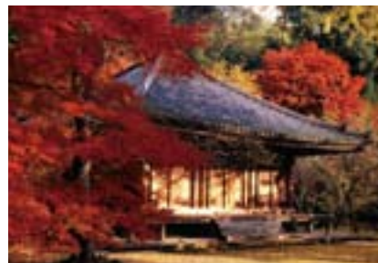
The great hall of Fukiji Temple is a national treasure. It is the oldest surviving timber structure in Kyushu.
