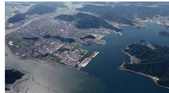
Saiki Port (Mejima East Berth and West Berth, from left)
