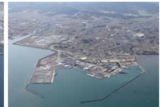
Nakatsu Port (East Berth1/2/3 and Chuo Berth, from left)
