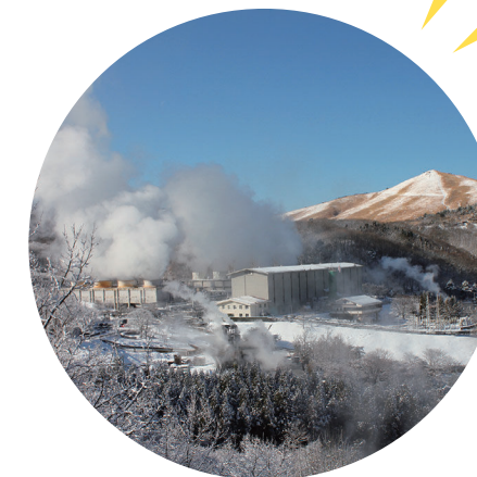
"Hachobaru Power Plant" uses steam from underground bedrocks and has garnered attention as the future of energy.
