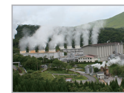
Hachobaru Power Plant (Learn about Geothermal Energy)
