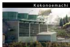
Kokonoemachi Hacchobaru Electric Power Plant 八丁原地熱発電所
